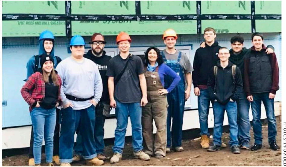
Ulster BOCES students work with Saugerties counselor Mike Catalano, fifth from right; Ulster BOCES teaching assistant Michelle Rosu, center; and Ulster BOCES Electrical Construction instructor Bob Jones, fourth from left.
